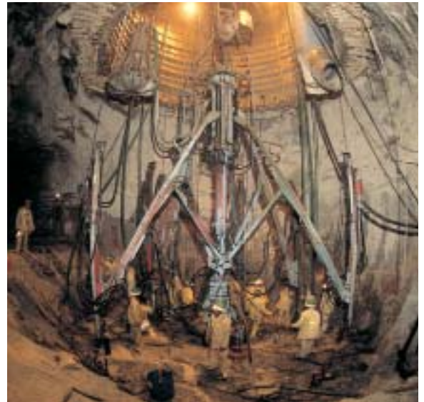
Shaft sinking and equipping
